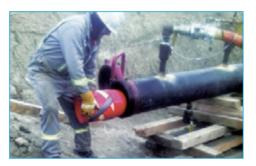
Pigging is a process that cleans and removes debris on the inside of the pipe using a device called a pig that's propelled through the pipeline by the normal water flow. Pigs are usually cylindrical or spherical to aid movement and cleaning efficiency.
